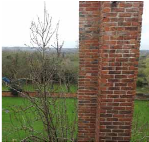
Plate 3: View from 2nd floor, Gorcott Hall
