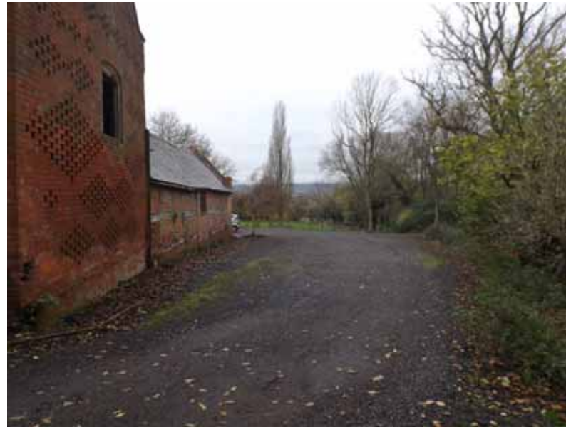
Plate 20: View looking west along access drive
