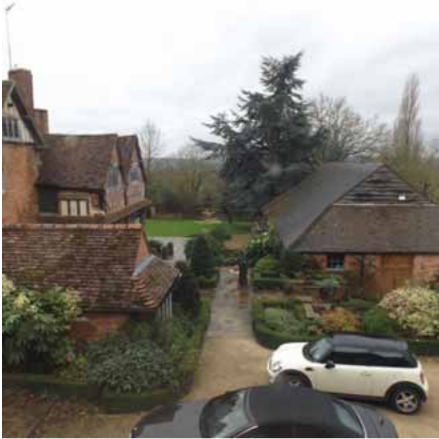
Plate 5: View from 2nd floor, Gorcott Hall
