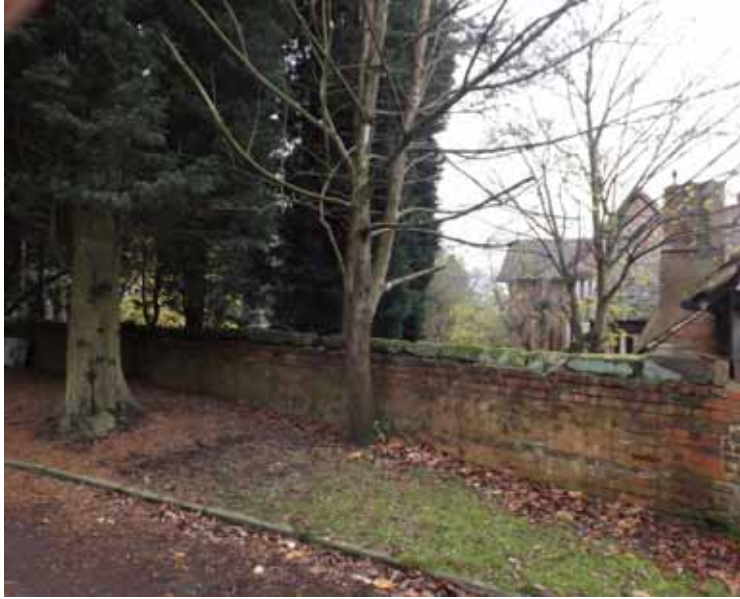
Plate 22: View of Hall from access drive
