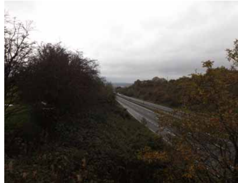
Plate 59: View from road bridge looking toward Hall and site
