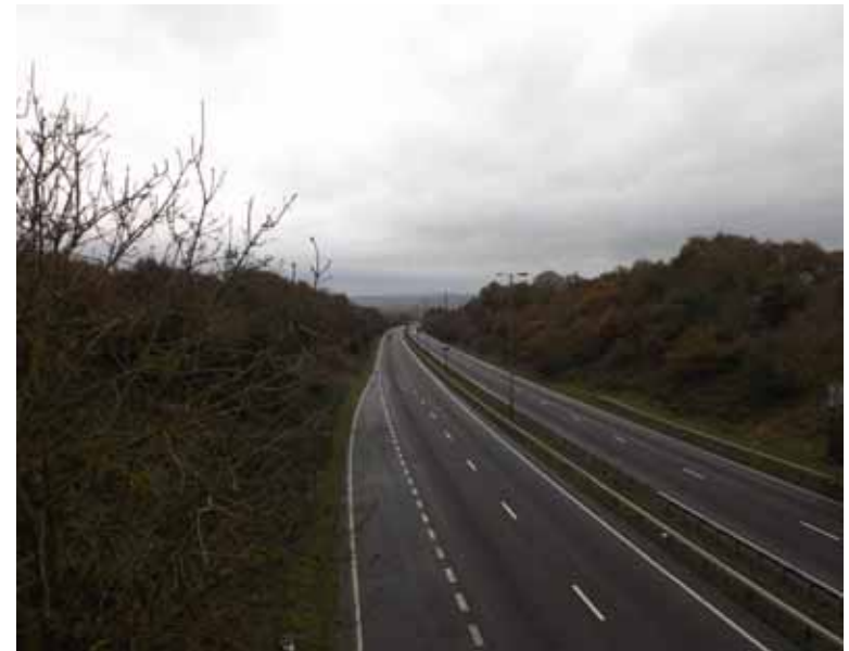
Plate 61: View from road bridge looking toward Hall and site
